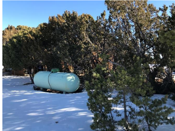
Picture 5: Low growing canopy over propane tank which can generate needle accumulation.
